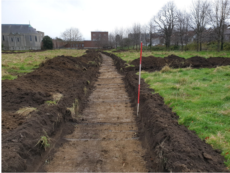
Plate 5: From NE, trench No. 6
